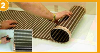
Roll out the ECOFILM<sup>SET</sup> elements and trim to length along the cutting line as required.
