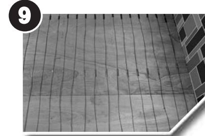
Ensure cable is laid in parallel lines
