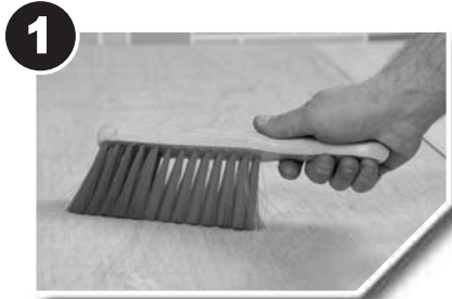
Ensure floor is clean & dust free
