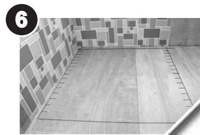
Mark perimeter & cable spacing
