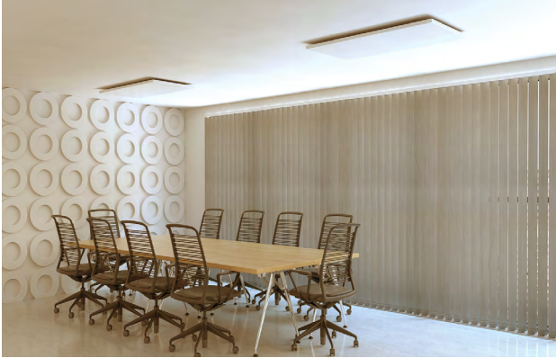
Ceiling mounted UB infrared panels
