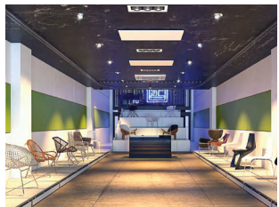
Ceiling mounted U+ infrared heating panels
